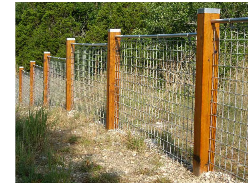
4' Hog wire and wood fencing
